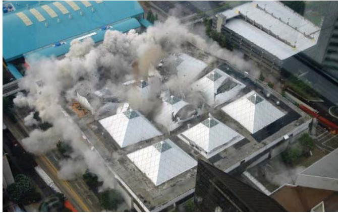
The 2010 Vision Plan identified the former Convention Center site as one of the most significant redevelopment parcels in Uptown, and was subsequently demolished.
